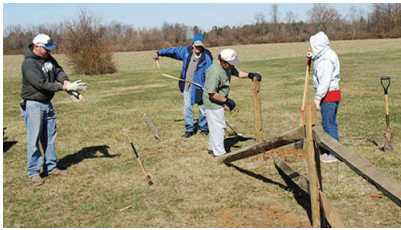
New fence at Heli area
